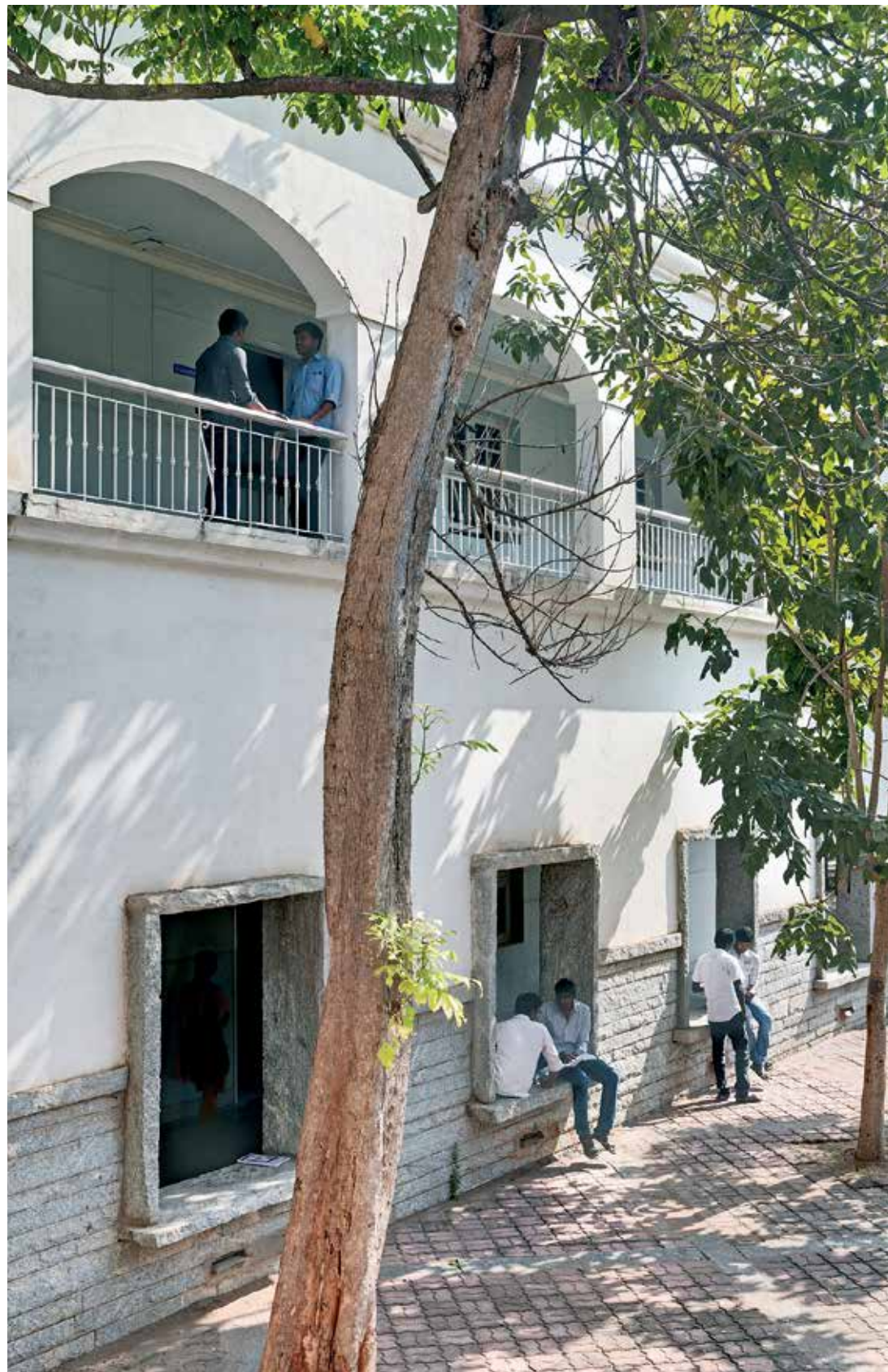
Left: the lower parts of building's walls are clad in stone, while arches open up the verandahs on the floor above
