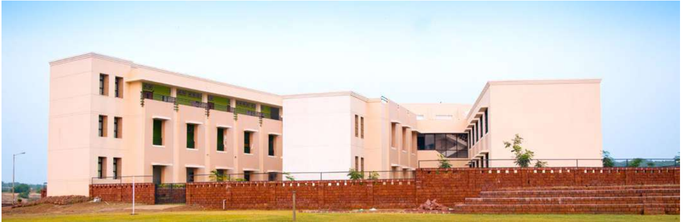
↑ Minimal openings on the south shield the classrooms from heat gain.
