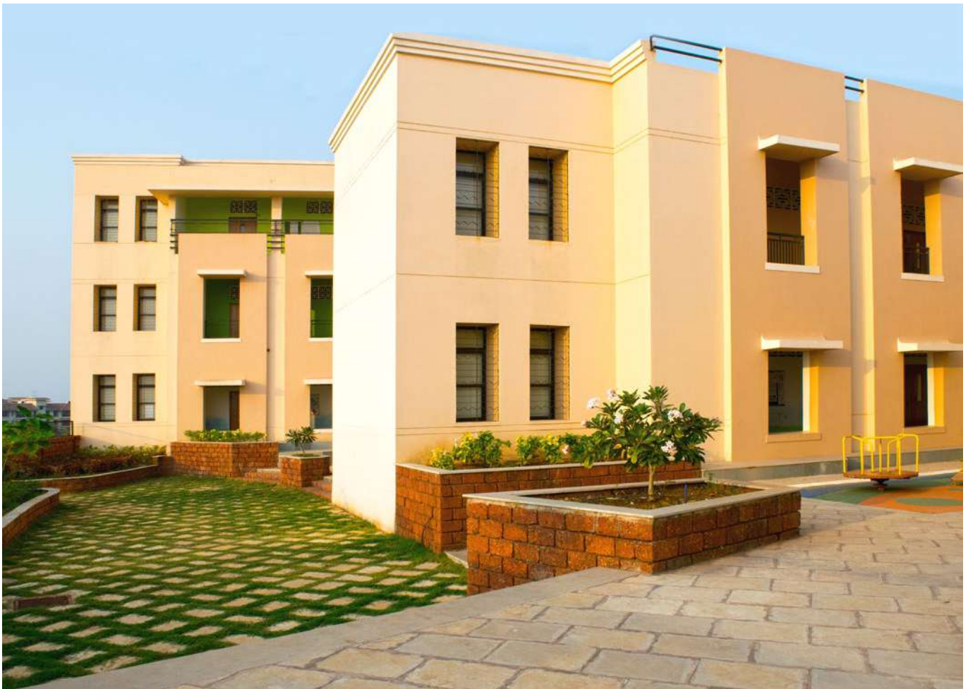
↑ Every classroom adjoins a landscaped courtyard.
