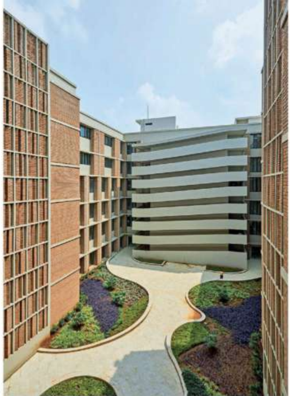
SUHRC 2019: Ventilation across the buildings to allow how increased rate of air circulation
