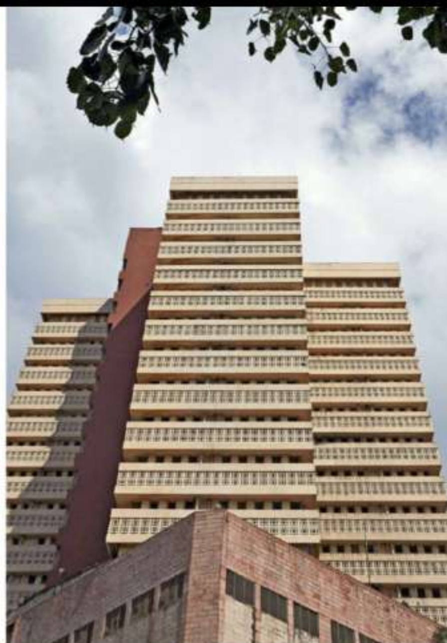
Hinduja Hospital 1980: Designed with large spans on the lower floors to allow for flexible use of spa
