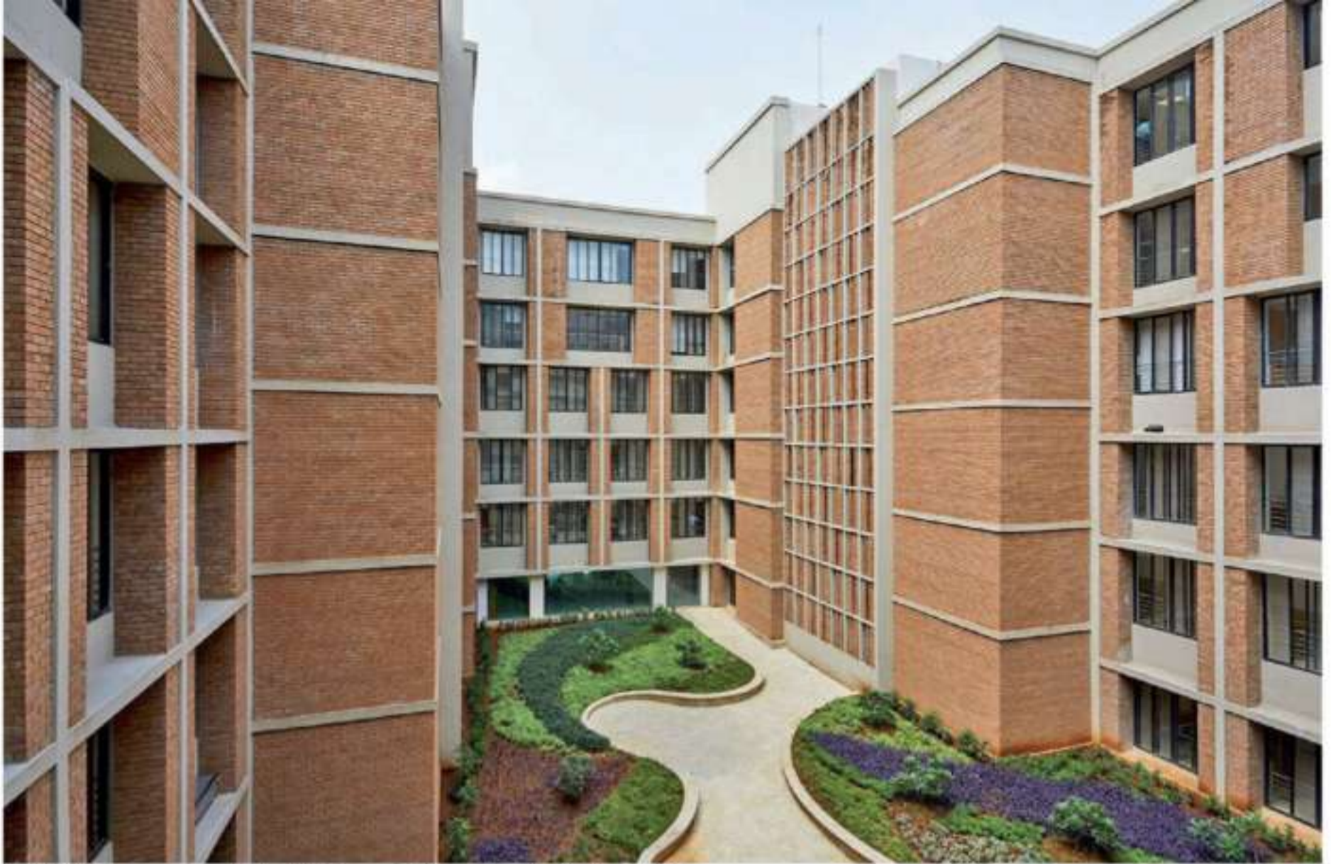
SUHRC 2019: Large courtyards in the building create buffer zones and naturally ventilated areas
