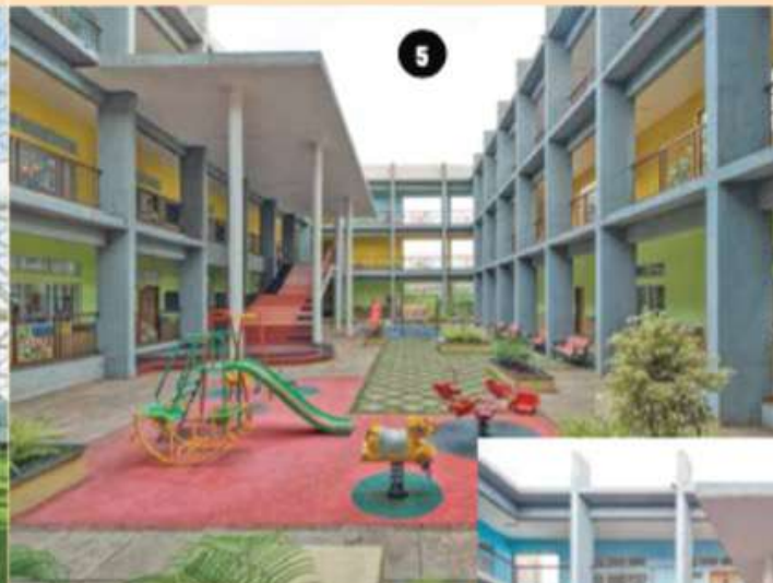
Fig 5-4: At the Jindal Vidya Mandir near Bellary, a central triple-height courtyard connects students across different levels to become a vibrant centre of activity. This visual connection fosters a sense of transparency between the indoors, outdoors and the landscape – creating a safe environment for interaction. © Hemant Patil.
