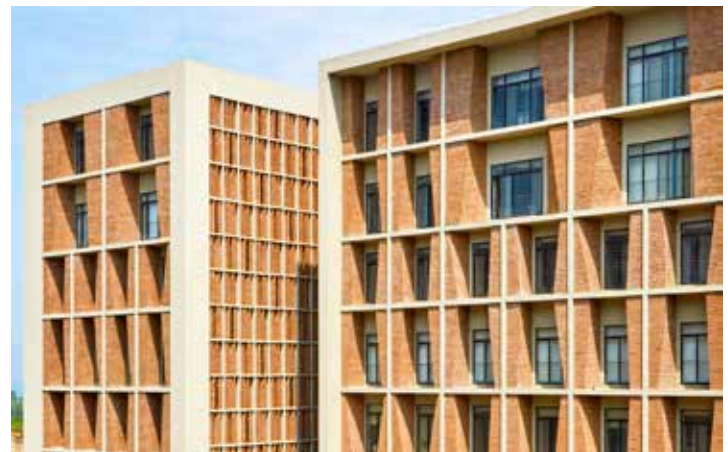
Figure 6(d): CEB jaali screens act as shading devices, SUHRC, Lavale, Pune (Photo Courtesy: Rajesh Vora)
