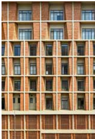
Figure 6(b): Twisted CEB boxing seen on the facade, SUHRC, Lavale, Pune (Photo Courtesy: Rajesh Vora)
