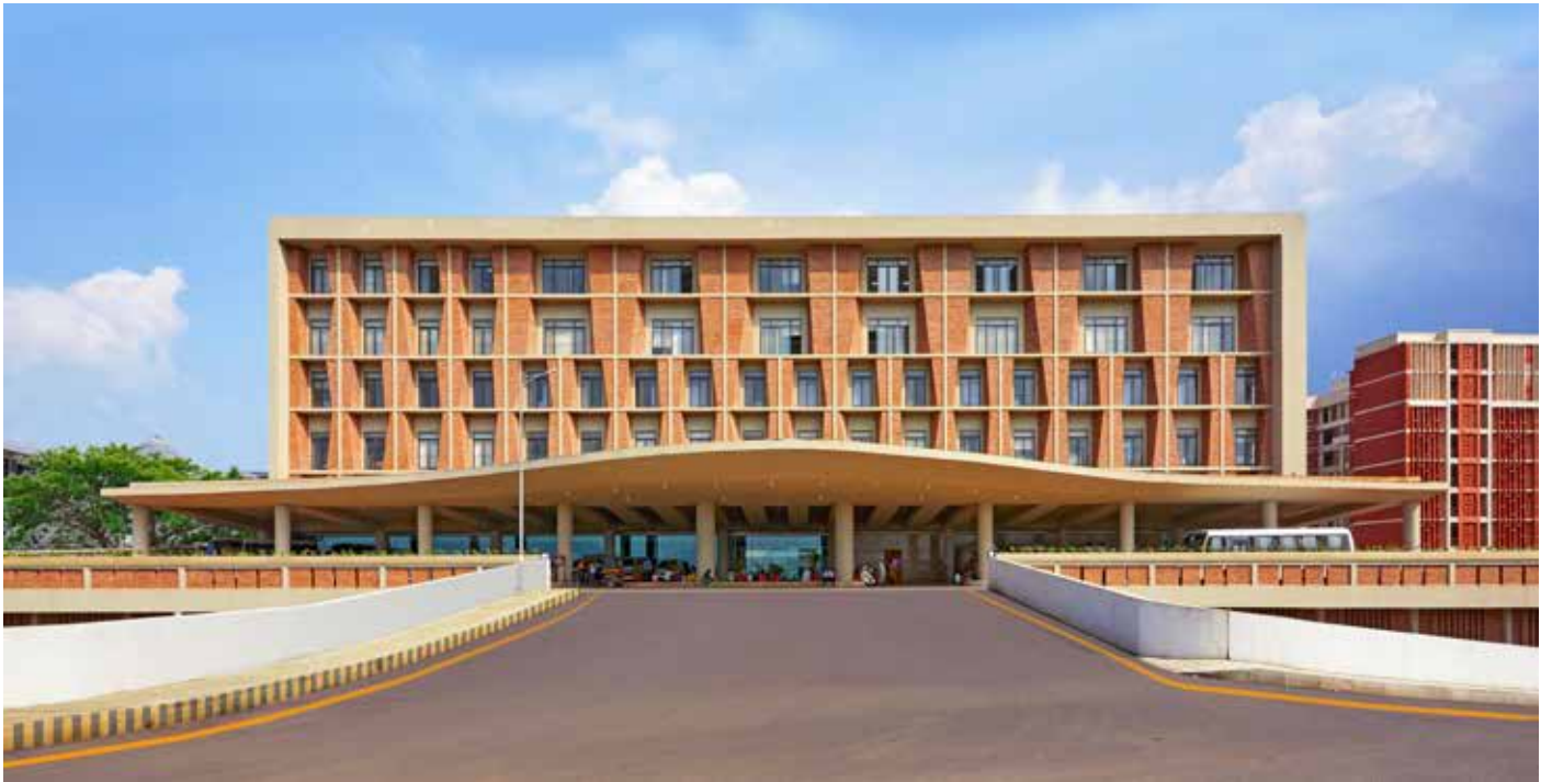
Figure 3: Curved roof shading the large entrance, SUHRC, Lavale, Pune (Photo Courtesy: Rajesh Vora)
