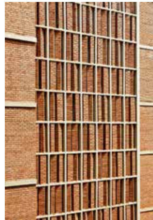
Figure 6(c): CEB jaali screens act as shading devices, SUHRC, Lavale, Pune (Photo Courtesy: Rajesh Vora)
