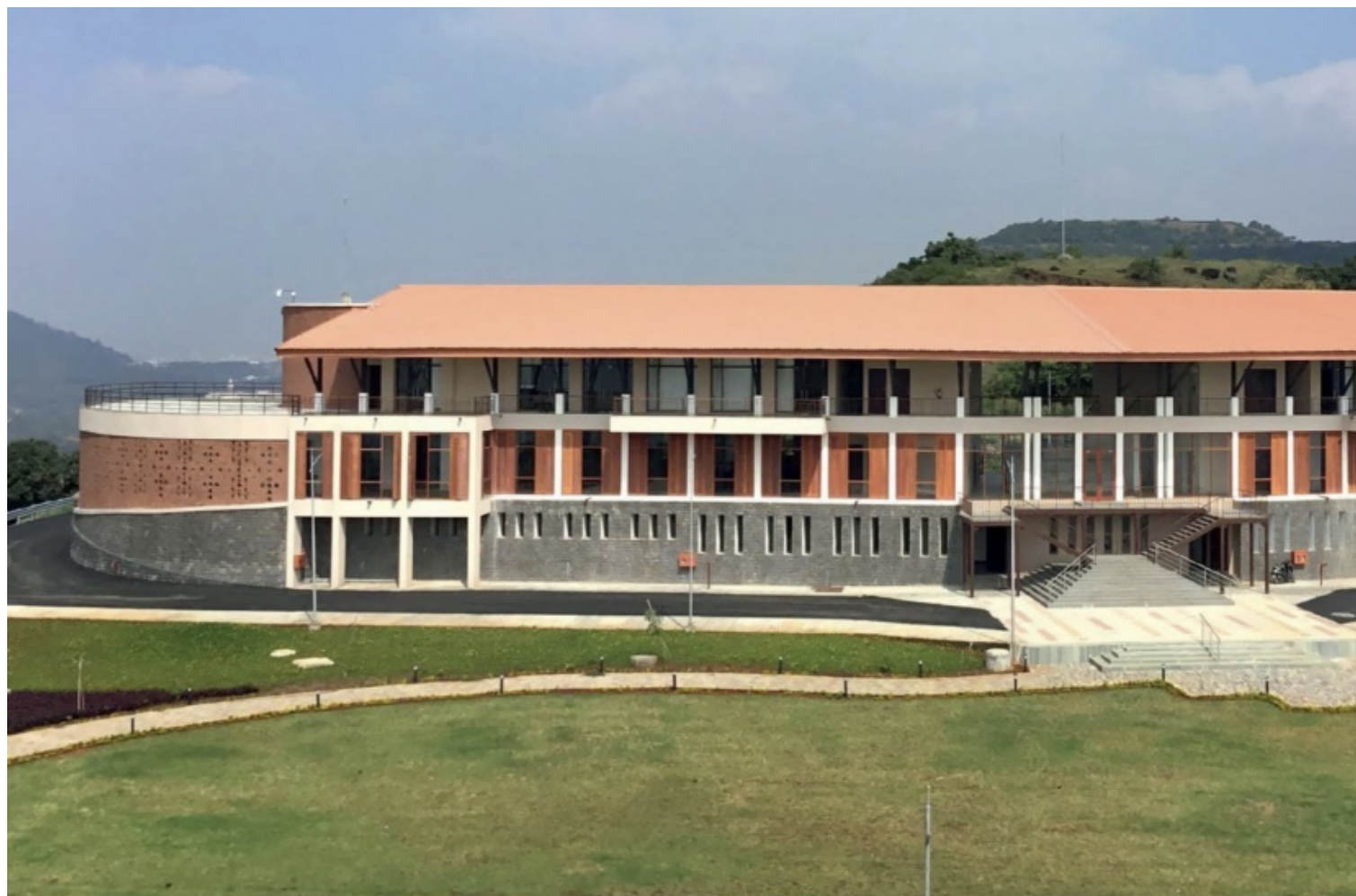
Symbiosis Sandipani, Lavale has been designed with 2.4m-wide single-loaded corridors, bringing the outside in, to ensure optimal ingress of daylight and fresh air
