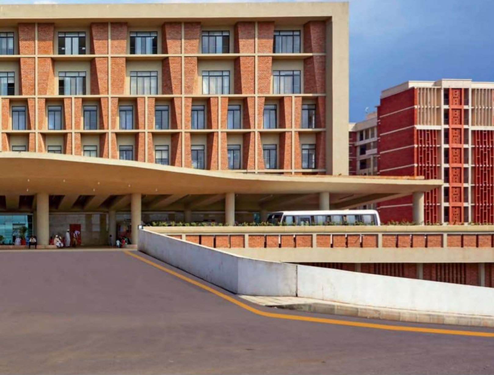
Entrance porch at SUHRC.
