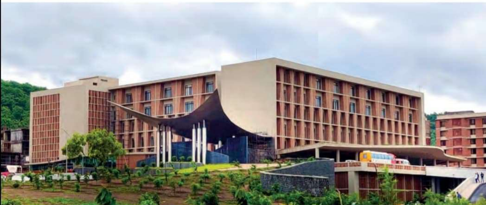
The entrance canopy for the Skill Centre draws inspiration from stainless steel surgical instruments.
